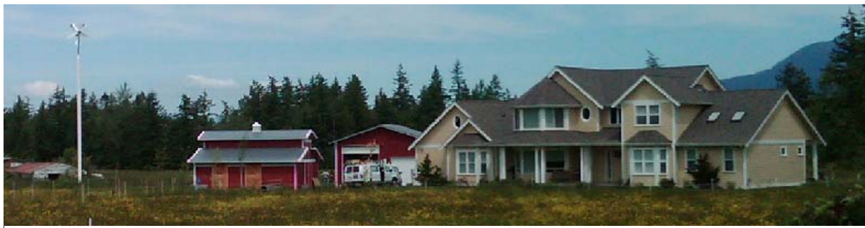
NWWP erects another V200 on June 8 th in a Seattle, Washington suburb.
